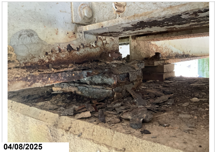
Span 2 Bent 3 Girder 2 active corrosion with flaking rust and section loss up to 1/16" and 1/4" section loss to bottom flange CS3 2 LF
