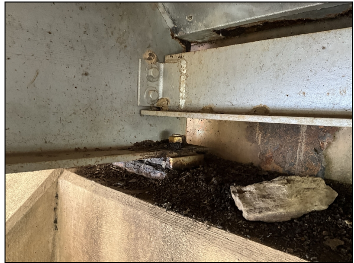
Beam ends could use a painting.
