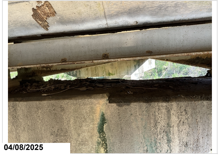
Typical dirt and debris on caps.
