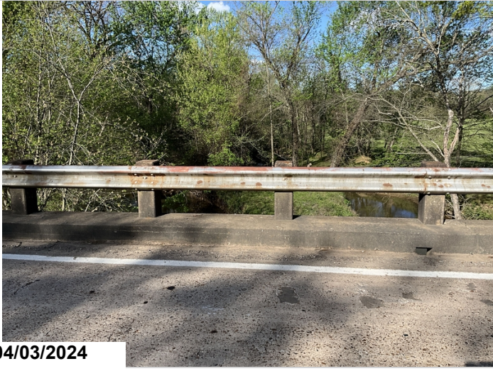
Typical paint failure on rail.
