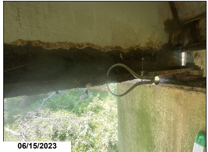
Span # 3, Girder 1 at bent 4-Section loss to bottom flange.
