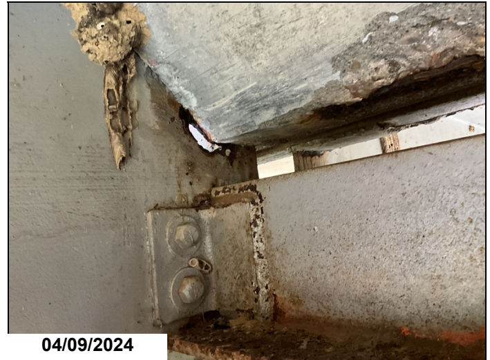
Span 3, bent 3, ahead side, girder 4, has a hole in the web at the haunch. CS3
