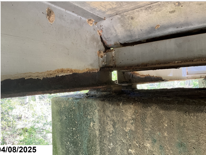
Span 1 Bent 1 Girder 1 Active corrosion with flaking rust typical on girder ends. CS3 8 LF
