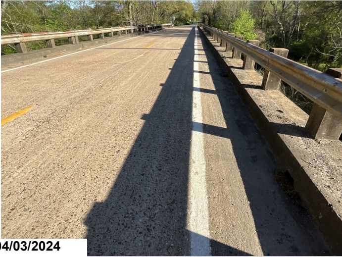
Dirt and debris in gutters
