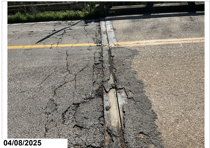
All joints have debris impaction. CS2 full length
