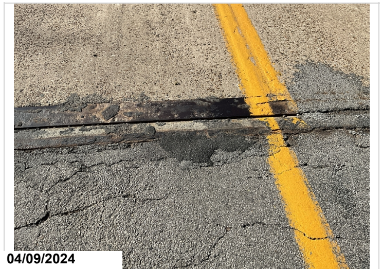
Typical debris impact in joints.
