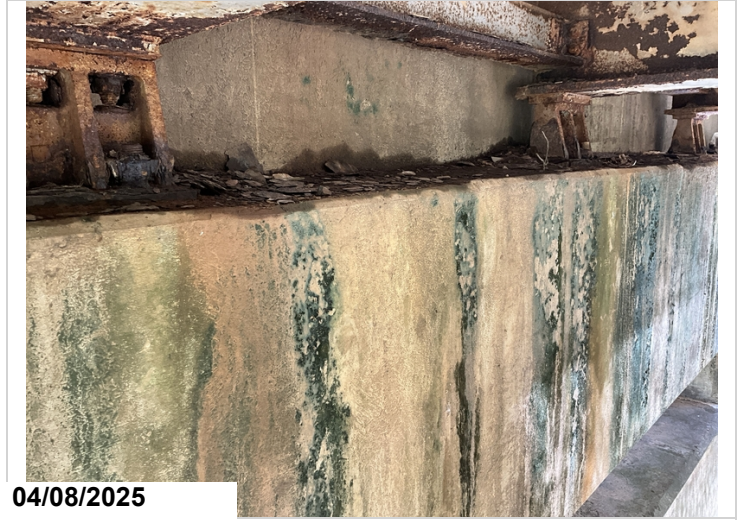
Span 4 Bent 5 fixed bearings have active corrosion with flaking rust. CS3 1 EA
