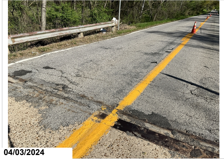
Joints need to be cleaned.
