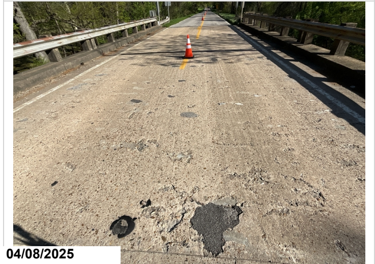
Span 4 Large areas of delamination. CS3 80SF
