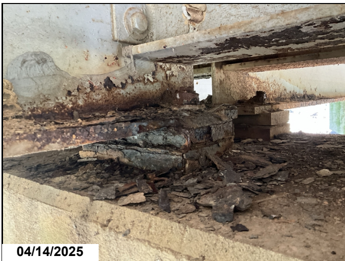
Span 2 Bent 3 Girder 2 active corrosion with flaking rust and section loss up to 1/16" and 1/4" section loss to bottom flange CS3 2 LF
