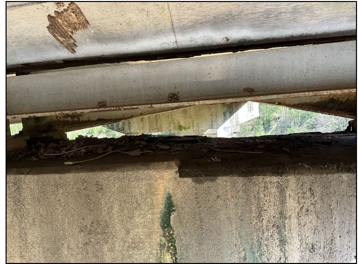
Typical dirt and debris on caps.
