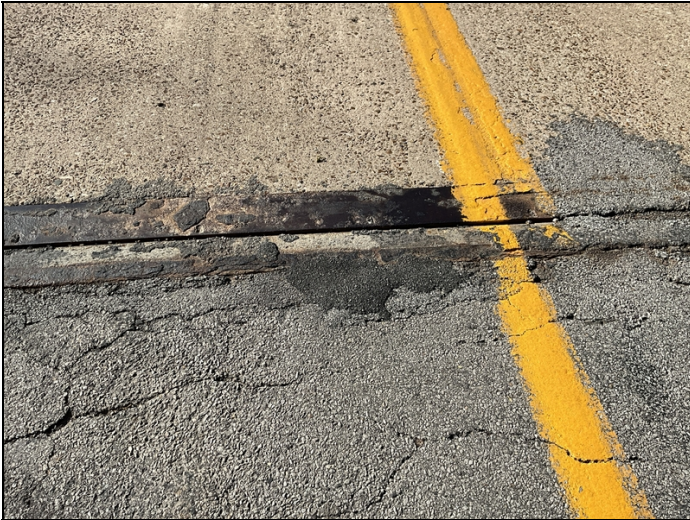
Typical debris impact in joints.
