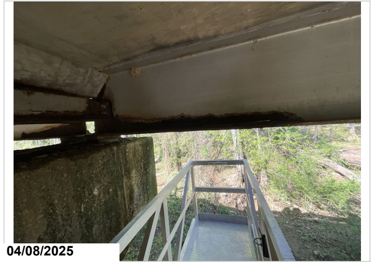
Span 2 Bent 2 Girder active corrosion with flaking rust and section loss up to 1/16" CS3 8 LF
