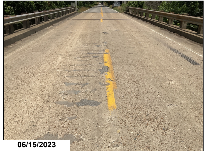
Span 4-Spall with exposed reinforcing steel
