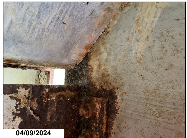
Span 3, bent 4, girder 5, has active corrosion and advanced section loss in haunch area. CS3 3/16"
