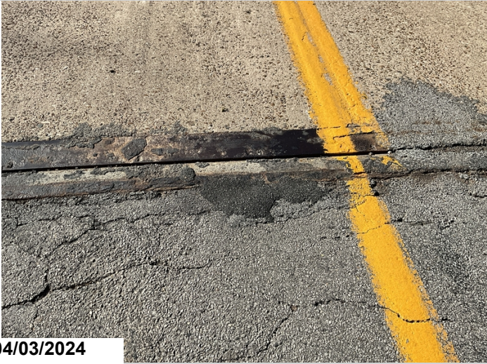
Typical debris impact in joints.
