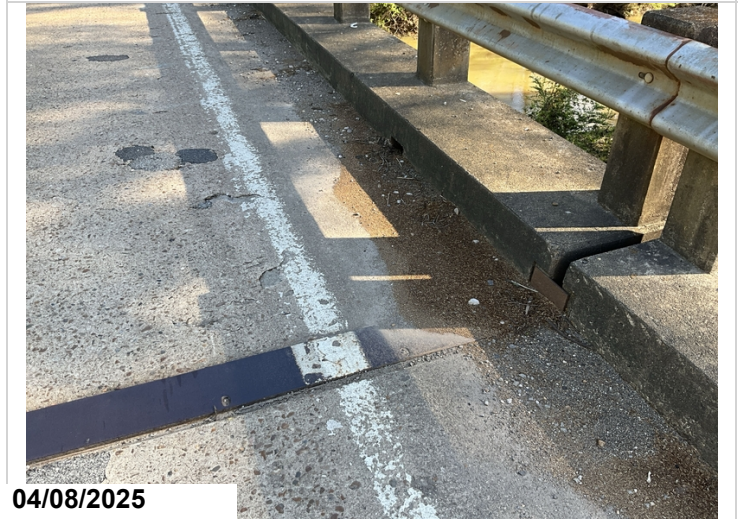
Typical debris restricts the deck drains.
