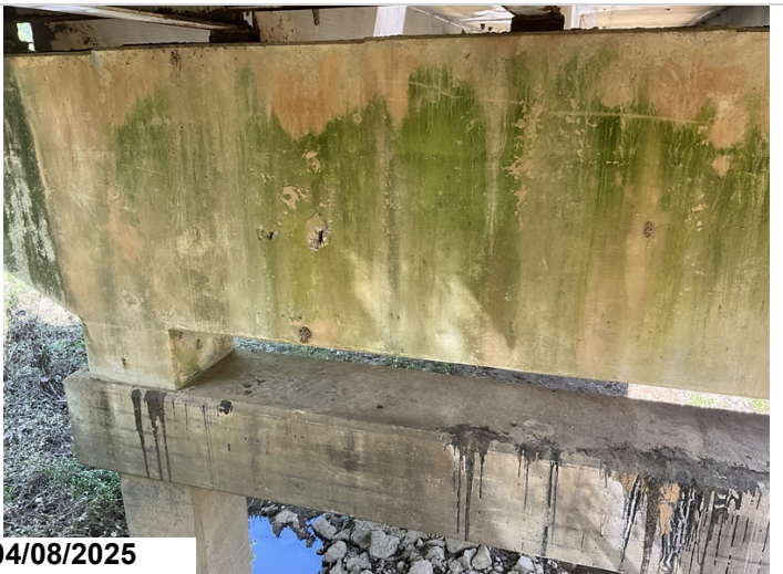
Span 3 Bent 4 Spalling with exposed reinforcing steel in face of cap. CS3 2 LF
