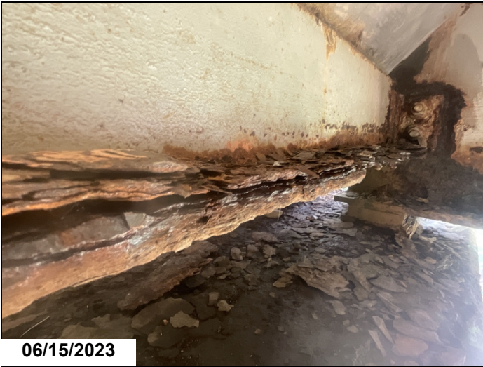
Span # 2, bay # 1-Section loss to diaphragm.
