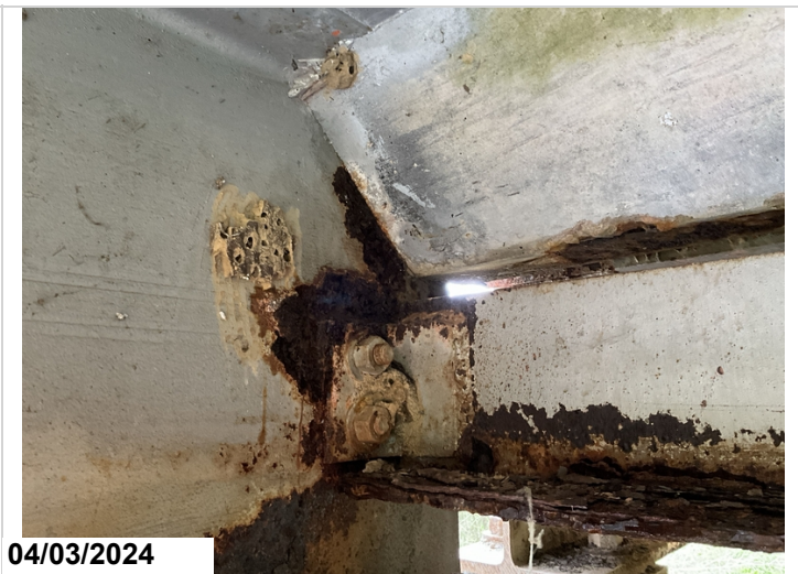
Span 3, bent 3, ahead side, girder 5, has active corrosion and advanced section loss in bottom flange. CS3 1/4
