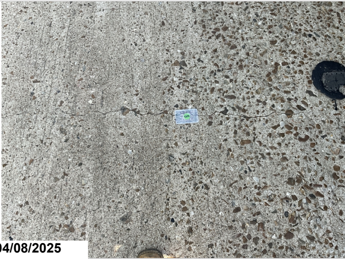
Span 1 left lane transverse cracking. CS3 .070 30 SF
