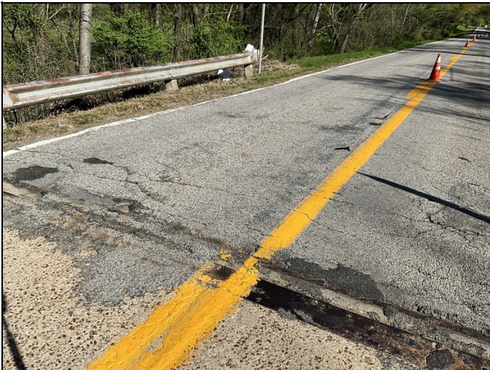
Joints need to be cleaned.
