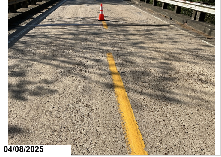
Typical wear in all spans.
