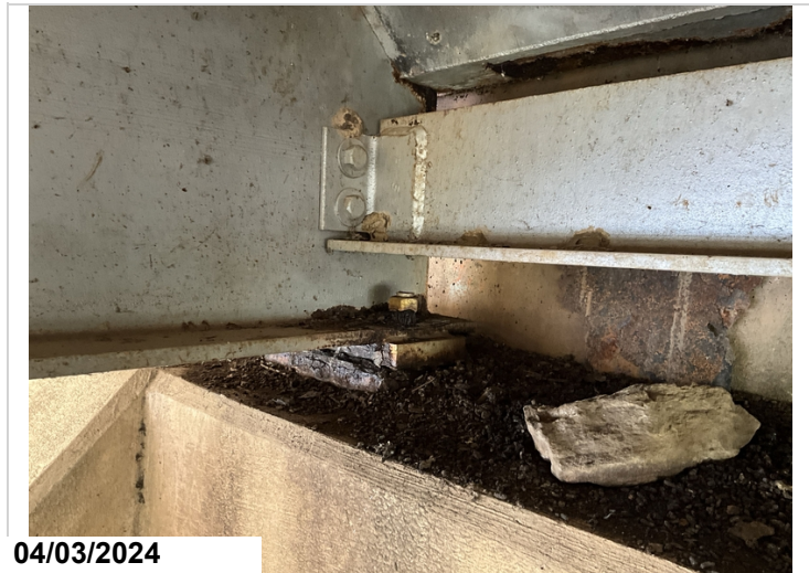
Beam ends could use a painting.
