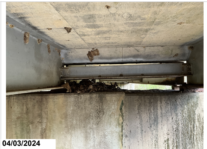
Caps have debris built up on top of them.
