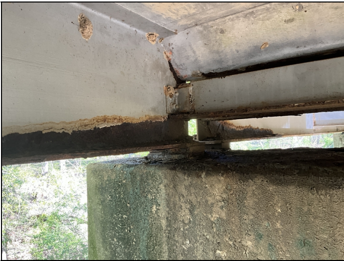
Span 1 Bent 1 Girder 1 Active corrosion with flaking rust typical on girder ends. CS3 8 LF
