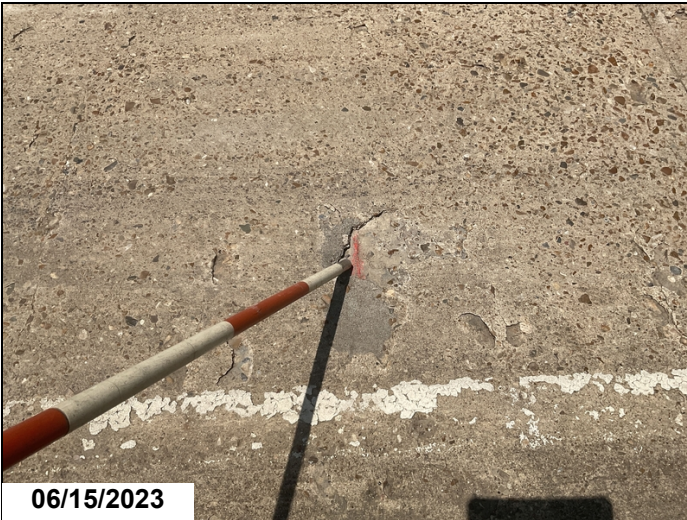
Span 4-Spall with exposed reinforcing steel
