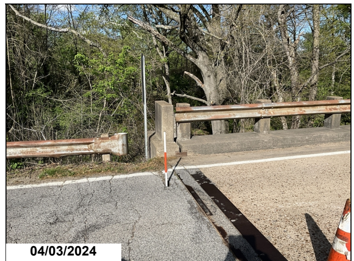
Abutment 1, approach, left lane, has settled. 2ft
