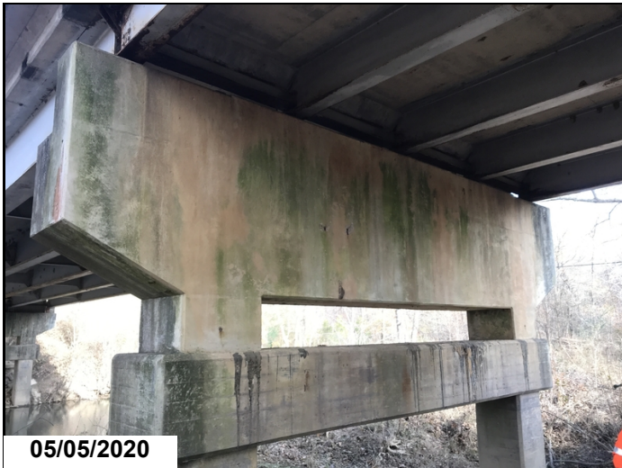
Bent # 4 cap-Spalling with exposed reinforcing steel.
