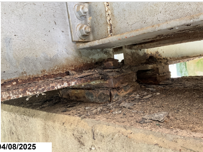
Span 2 Bent 3 Girder 3 active corrosion with flaking rust and section loss up to 1/16" and 1/4" section loss to bottom flange CS3 2 LF
