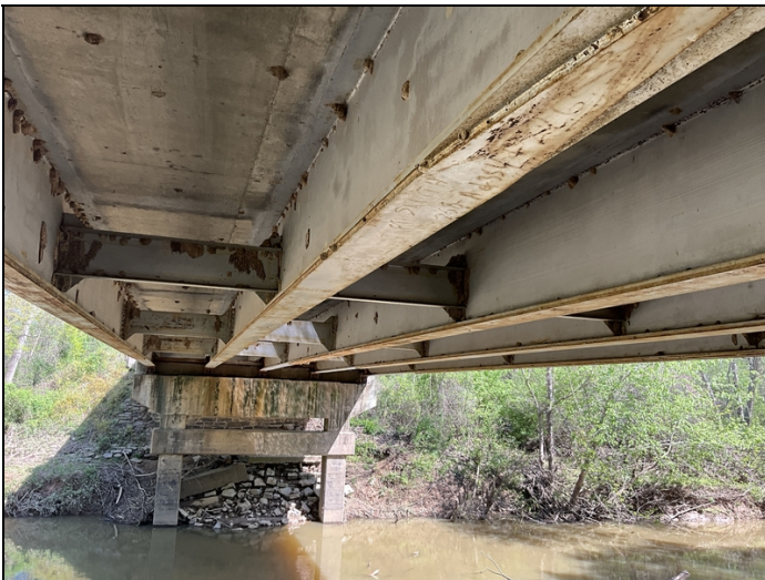
Girder have a failing paint system.
