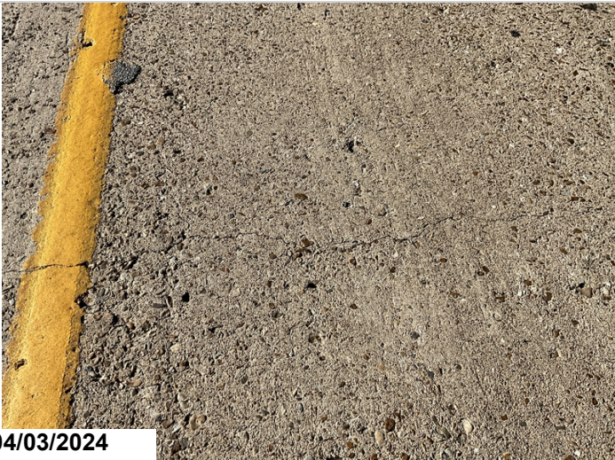
Sealable deck cracking
