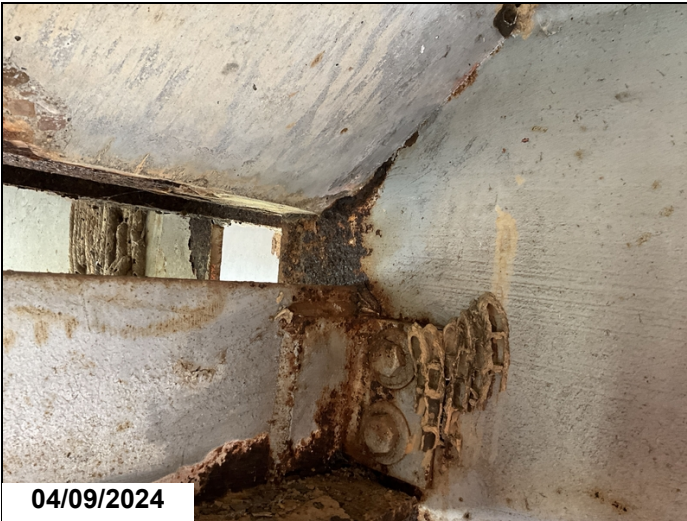
Span 3, bent 4, girder 4, has active corrosion and advanced section loss in haunch area. CS3 1/16
