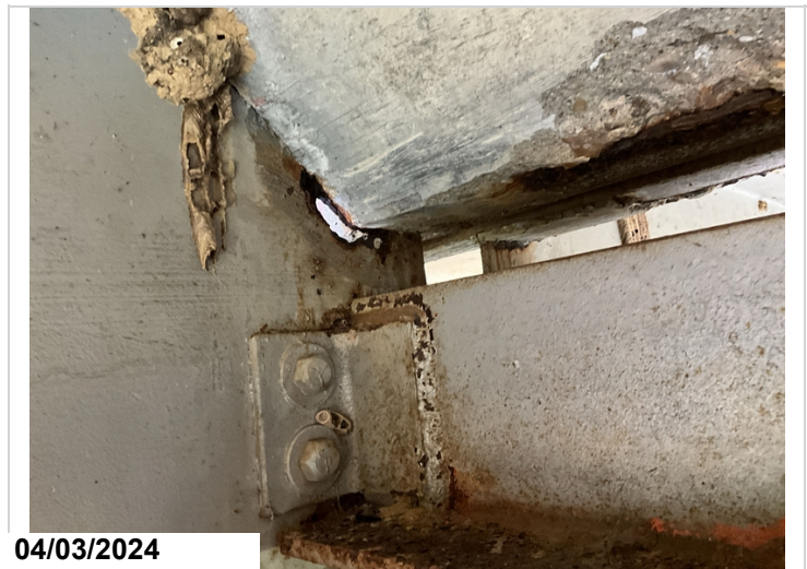
Span 3, bent 3, ahead side, girder 4, has a hole in the web at the haunch. CS3
