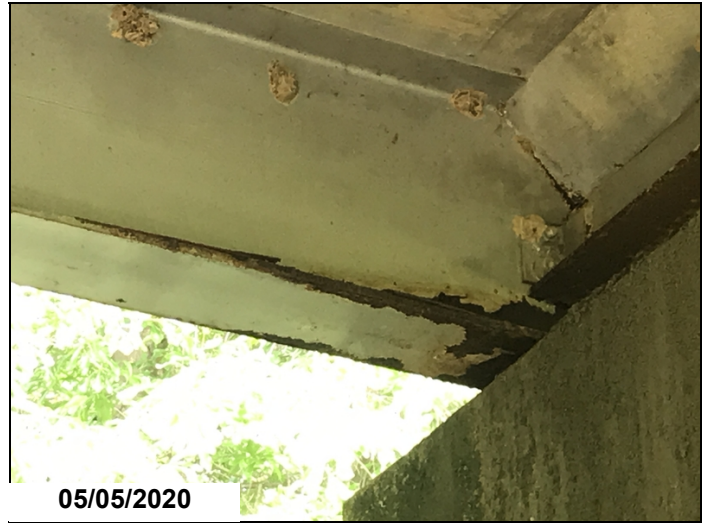
Beam # 1 at bent # 2-Active corrosion.
