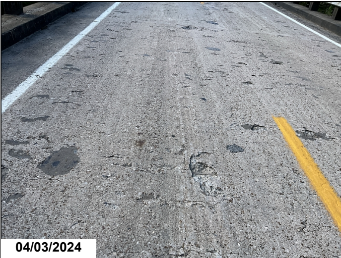
Span 4-Spall with exposed reinforcing steel
