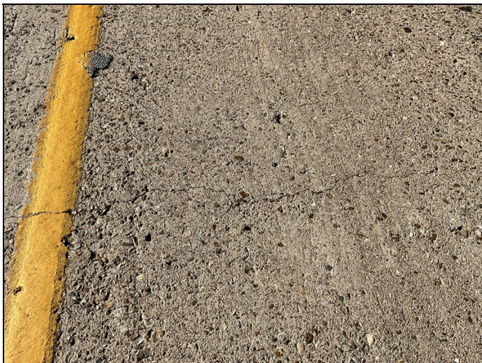
Sealable deck cracking
