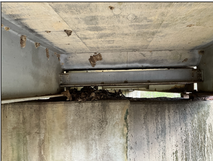
Caps have debris built up on top of them.
