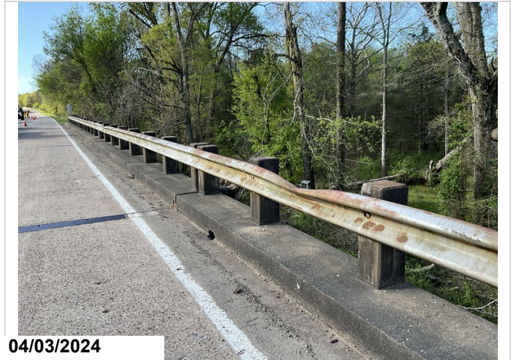
Spans 2, 3, and 4, left side, has damaged guard rail. 11 LF
