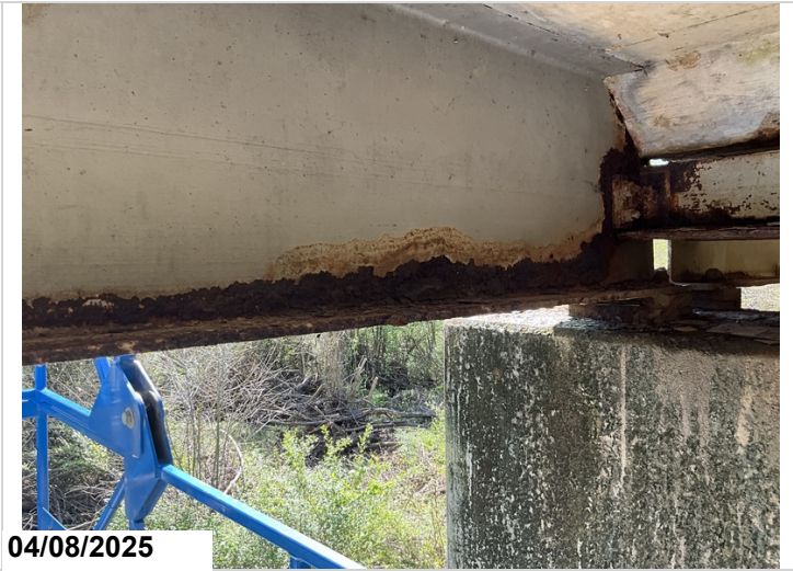
Span 2 Bent 2 Girder 5 active corrosion with flaking rust and section loss up to 1/16" CS3 8. LF
