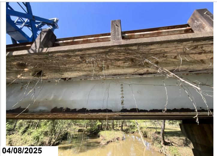
Span 4 Right edge of deck cracking with efflorescence. CS2 20 SF
