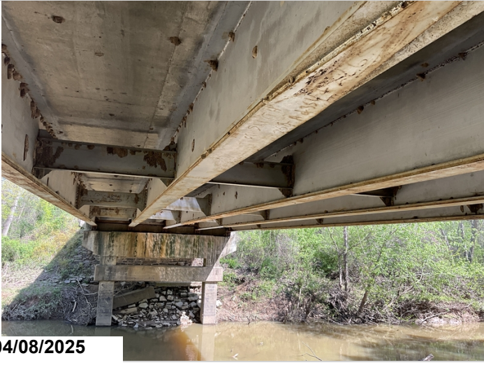
Girder have a failing paint system.
