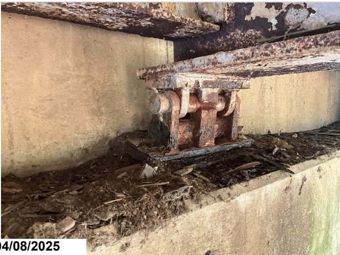
Span 4 Bent 4 Girder 2 Bearing fully extended at 60 degree CS3 1 EA
