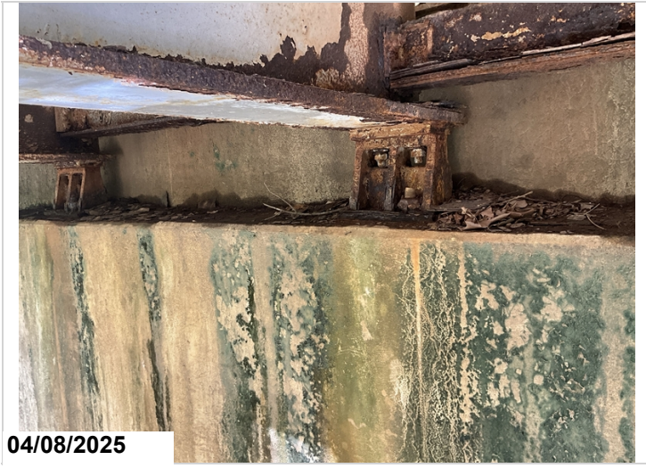
Typical debris on caps
