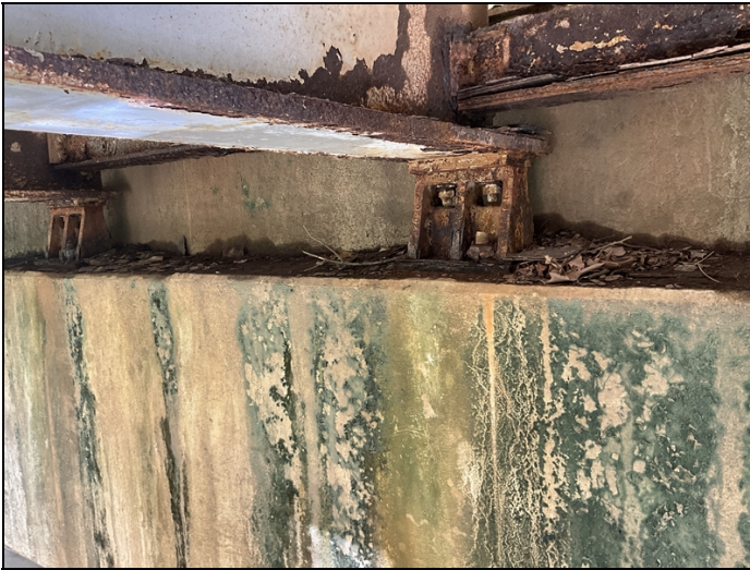
Typical debris on caps
