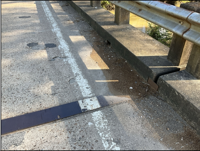
Typical debris restricts the deck drains.
