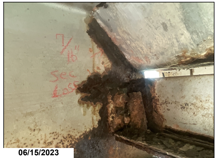
Span # 3, beam # 1 at bent # 4-Section loss to web at expansion dam and diaphragm connection.
