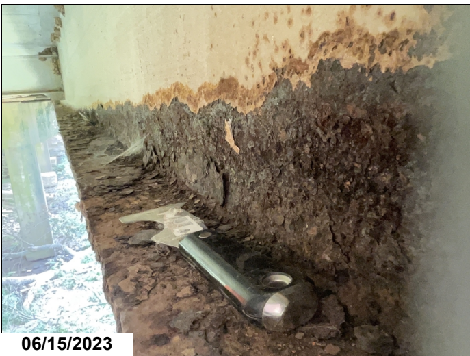
Span # 3, beam # 1 at bent # 4-Section loss to bottom flange.
