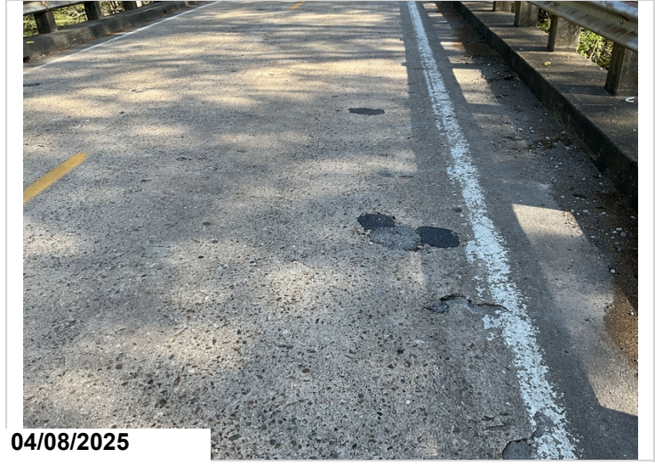
Span 4 Right lane large delaminated areas, potholes with temporary repairs. CS3 60 SF
