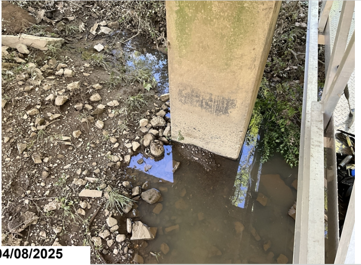
Span 3 Bent 3 Typical abrasion on all columns. CS2 1 EA
