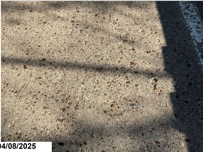
Typical map cracking in all spans.
