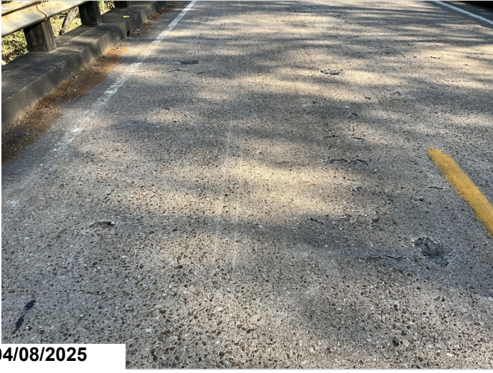
Span 4 Left lane large delaminated areas, potholes with temporary repairs. CS3 85 SF
