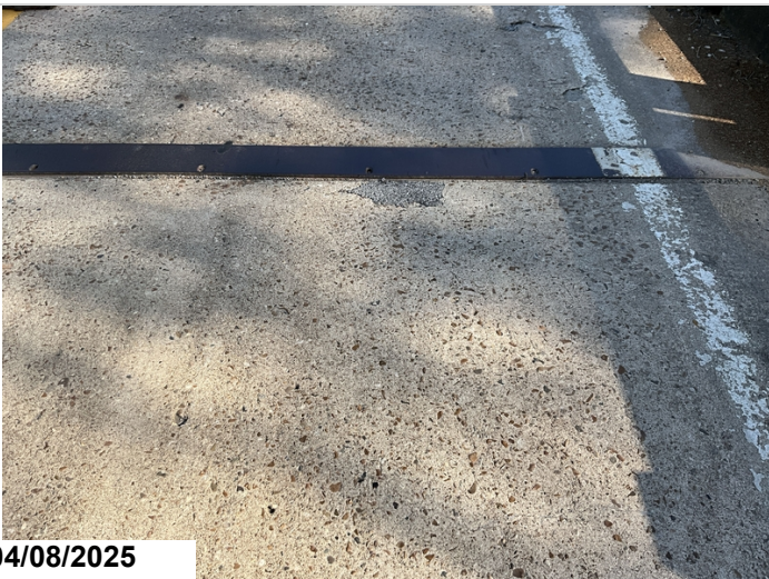
Span 3 Right lane right wheel paths spalling. CS3 2 SF
