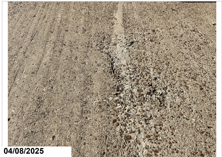
Span 2 Right lane delaminated area. CS3 8 SF
