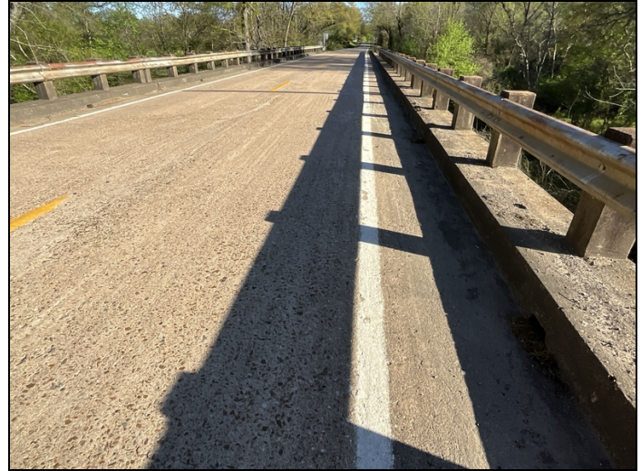
Dirt and debris in gutters
