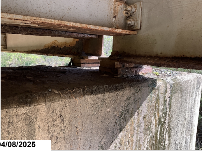
Span 1 Bent 1 Girder 5 Bearing has active corrosion with flaking rust. CS3 1 EA
