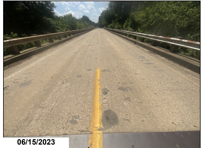
Span 4-Numerous spalls / delaminated areas
