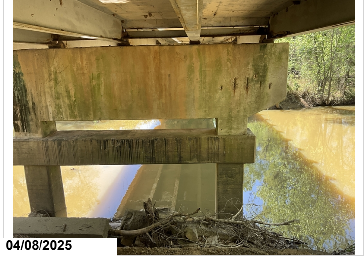
Span 5 Bent 5 Spalling with exposed reinforcing steel. CS3 4 LF
