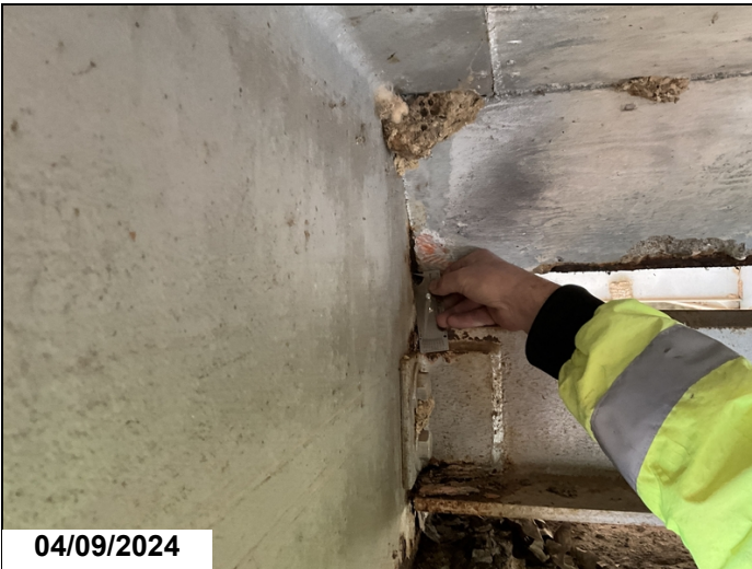
Span 2, bent 2, ahead side, girder 4, has active corrosion in haunch area with section loss. CS3 1 LF
