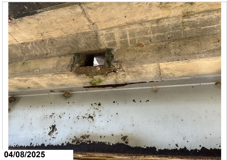
Span 3 Right spalling in the deck drain. CS2 2 SF
