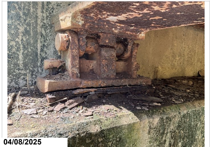
Span 4 Bent 4 Girder 5 Active corrosion with pack rust. CS3 1 EA
