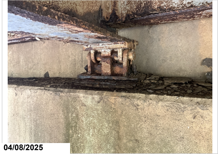
Span 4 Bent 4 Girder 3 Active corrosion with flaking rust. CS3 1 EA
