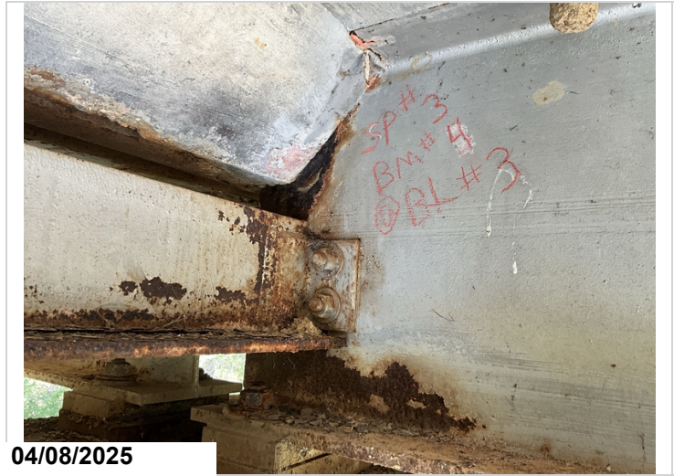
Span 3 Bent 3 Girder 4 active corrosion with flaking rust and advanced section loss 4" hole in web CS3 2 LF
